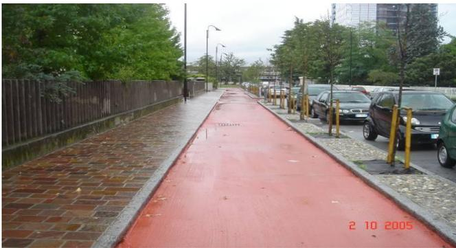
**3C PHOTOCATALYTIC PAVEMENT** can have a rough or smooth surface.
